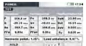
Detailed Power Measurements at Phase L1
